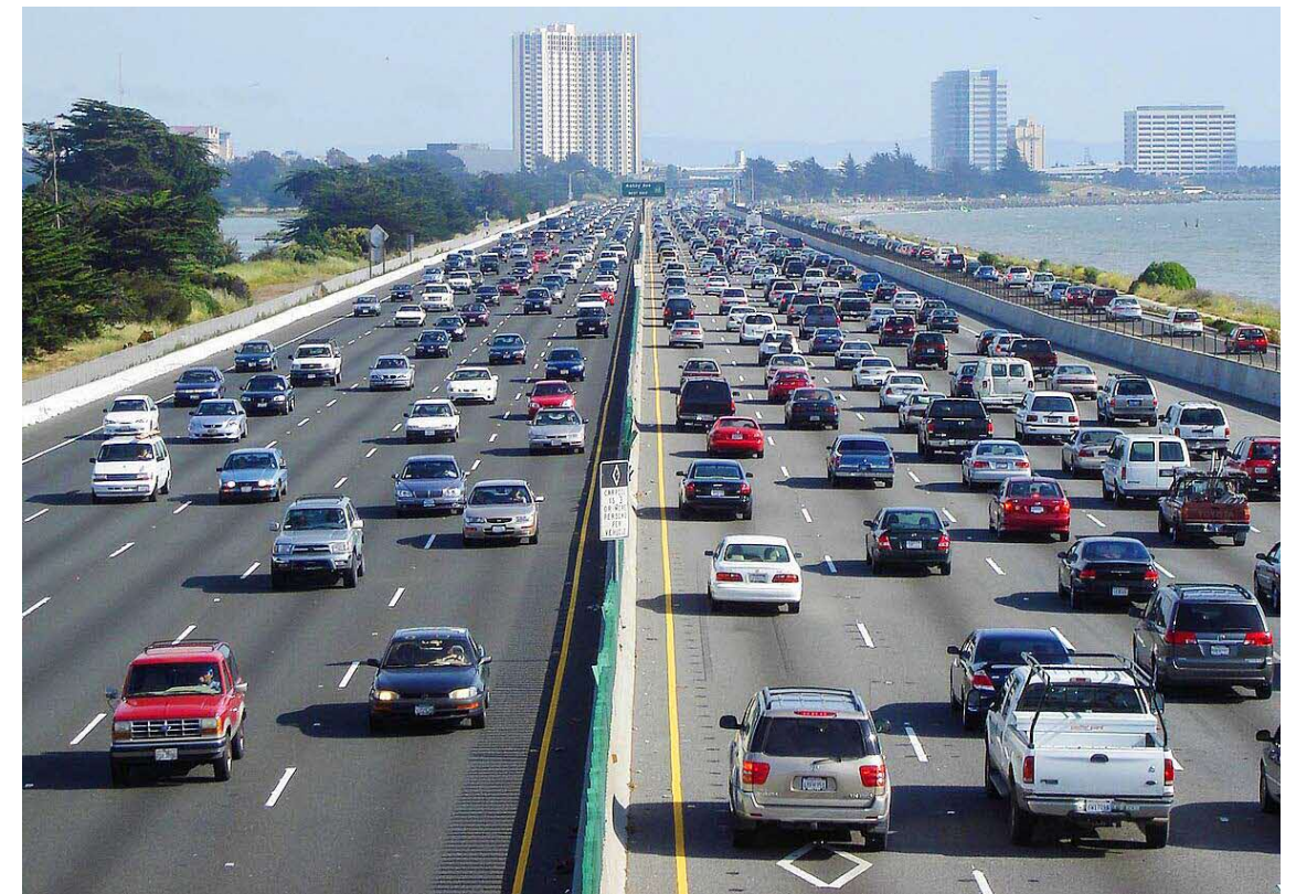
Interstate 80 in California. Transport assessments that focus on vehicle capacity can continue to perpetuate car-centric infrastructure such as multi-lane freeways, while overlooking liveability outcomes such as safety, comfort and vibrant public spaces.
